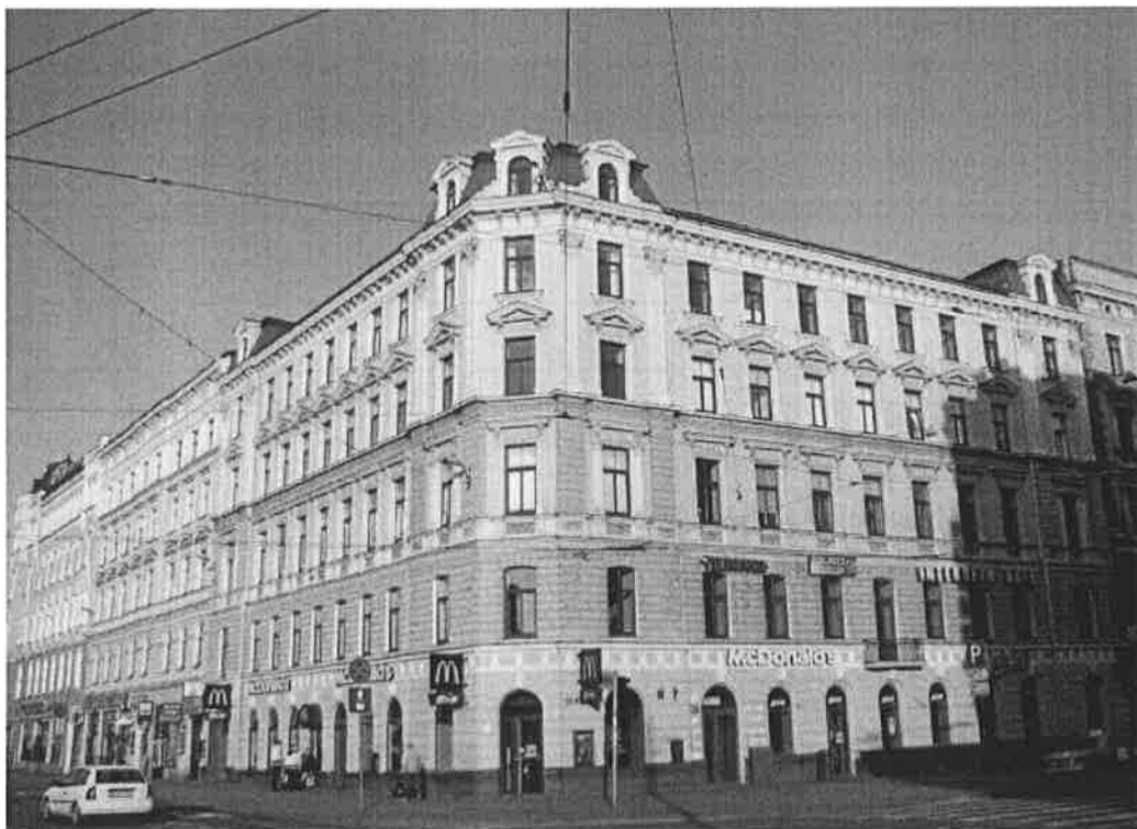
Commercial & office building – Merkela Street, Riga, Latvia
