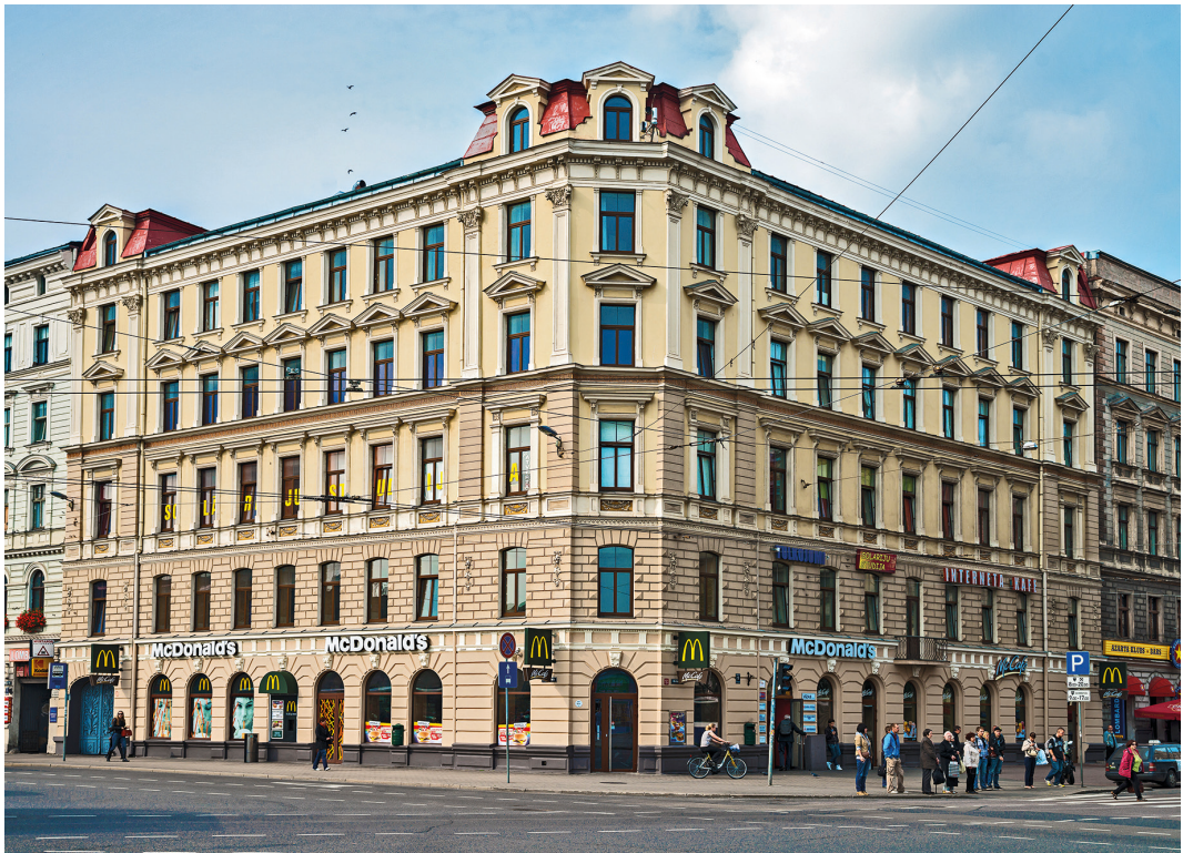
Commercial & office building – Merkela Street, Riga, Latvia
