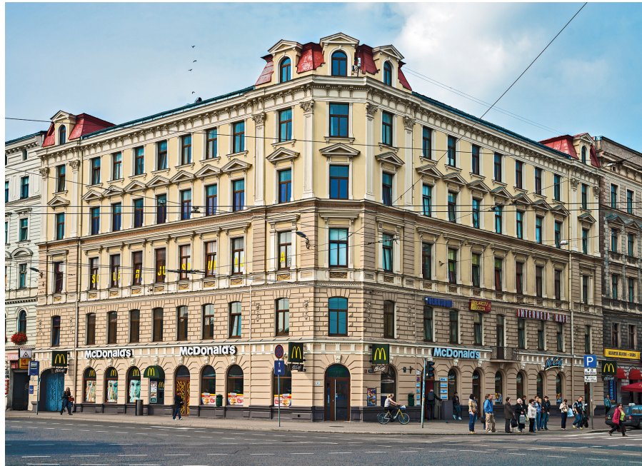
Commercial & office building – Merkela Street, Riga, Latvia
