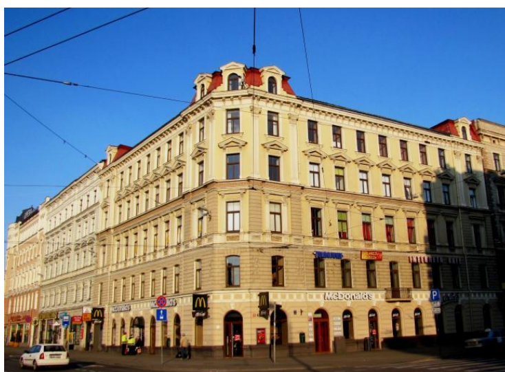
Commercial & office building – Merkela Street, Riga, Latvia
