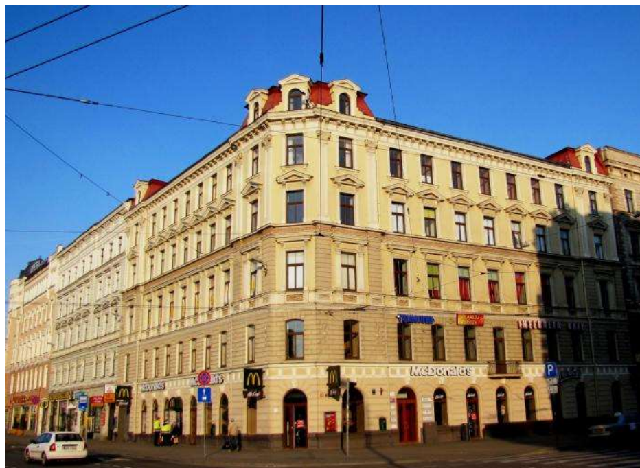
Commercial & office building – Merkela Street, Riga, Latvia
