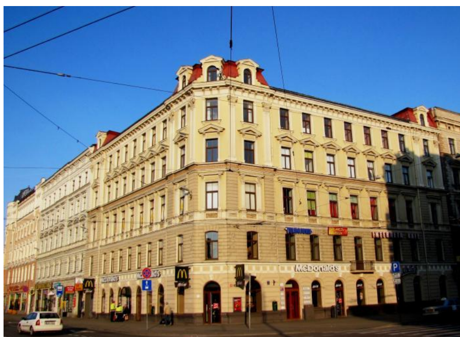
Commercial & office building – Merkela Street, Riga, Latvia
